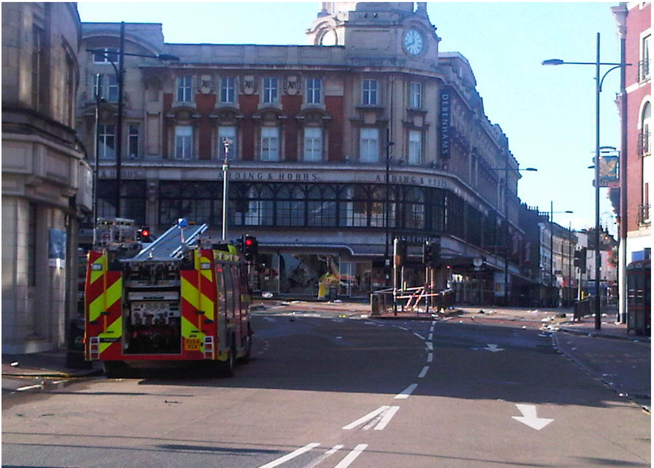
Clapham – photo taken this morning by Mike Jones, COO, showing damage to the Debenhams store
